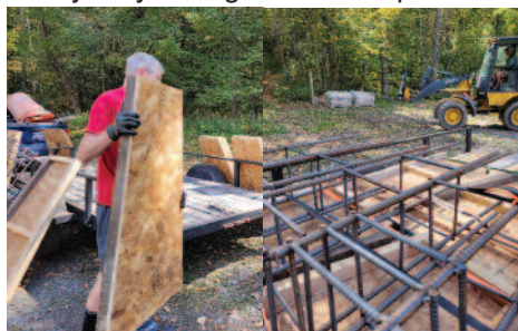
Material for footings, to go up the hill, 9/20/24
