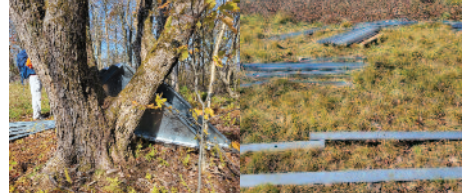
More parts and pieces awaiting a "lift", 10/18/24
