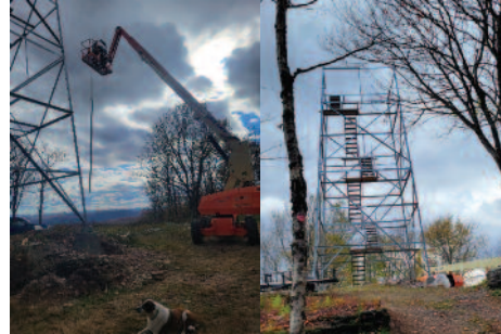
The tower was taking shape, 10/9/24
